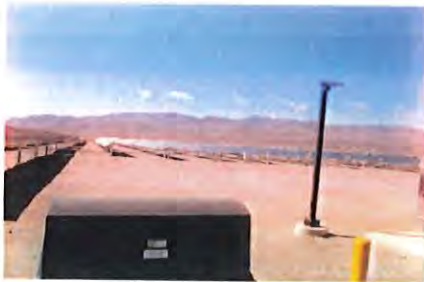
Luning Energy Solar Plant
