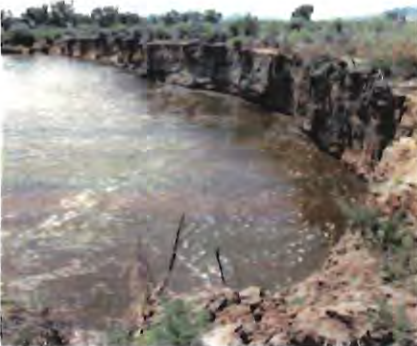
Mitchell Bank Stabilization
