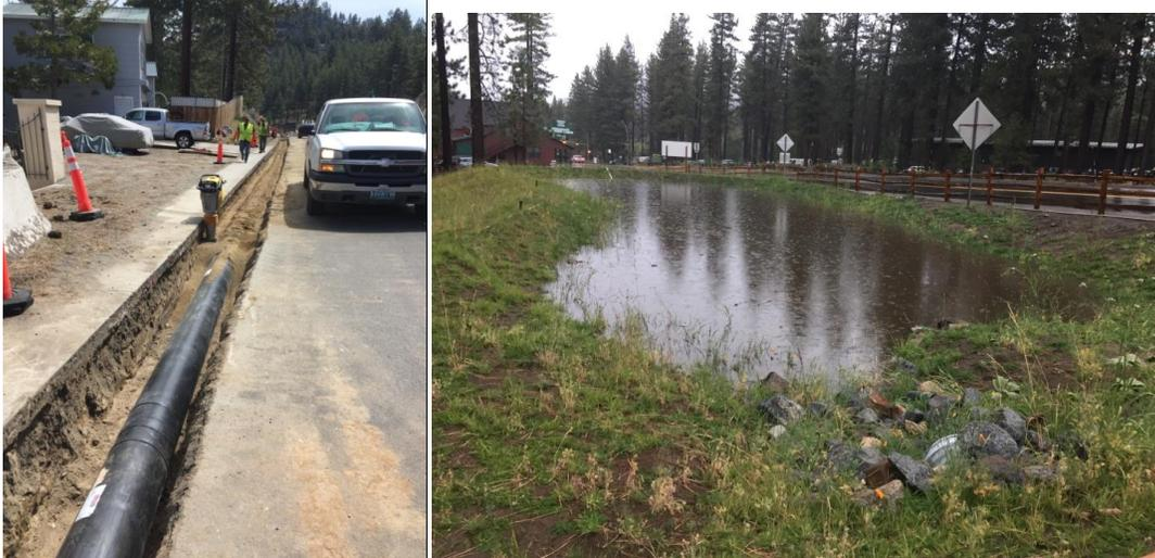
**Zephyr Cove GID Water Quality Improvement Project: Left, installation of storm drain, Right, Newly constructed basin collecting runoff.**
